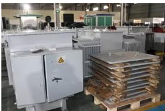
Oil Box Assembling
