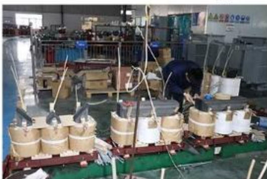
Iron Core Stacking
